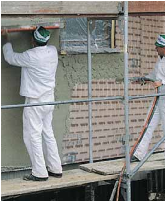
Mechanical application of Sto plaster using a PFT Ritmo mixing pump.
