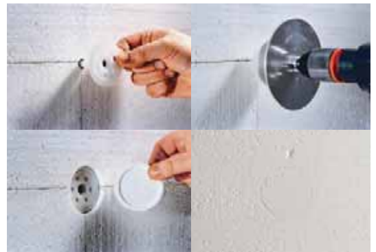
StoTherm Anchor installed on a masonry substrate.
