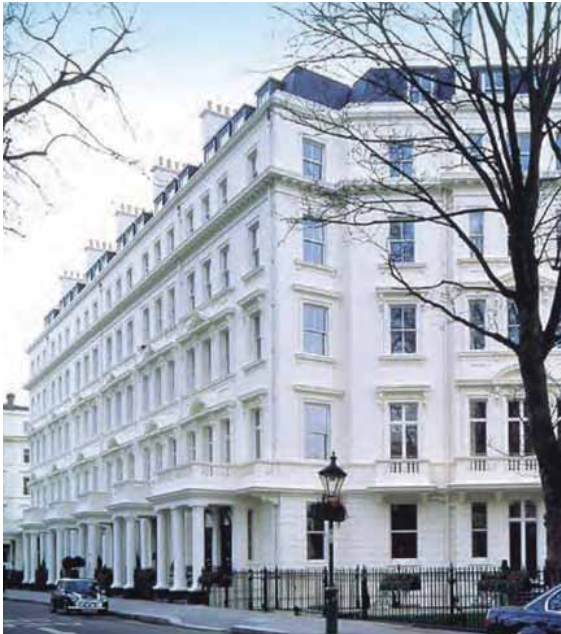
StoTherm Insulation System; Stanhope Gardens, London.
