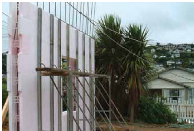
1. Step: setting of EPS blocks
