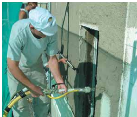
Step 2: application of the finishing render by a Sto applicator.
